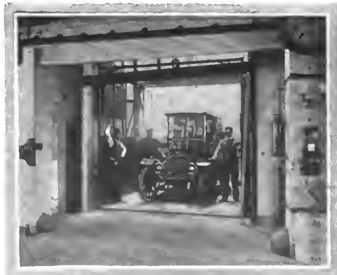
ONE OF THE HUGE ELECTRIC ELEVATORS.
